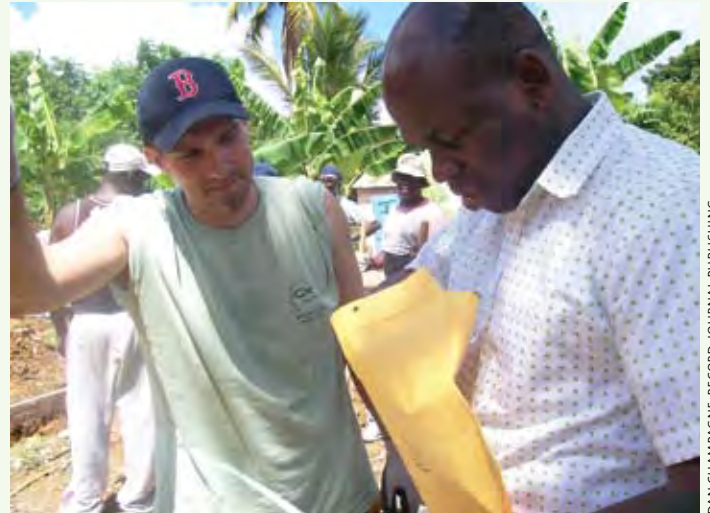
John Powers, YSN's Director of Public Affairs, goes over details with Moises Sifren, Administrator of the Good Samaritan Hospital, while building a school in a sugarcane village near La Romana, Dominican Republic.
