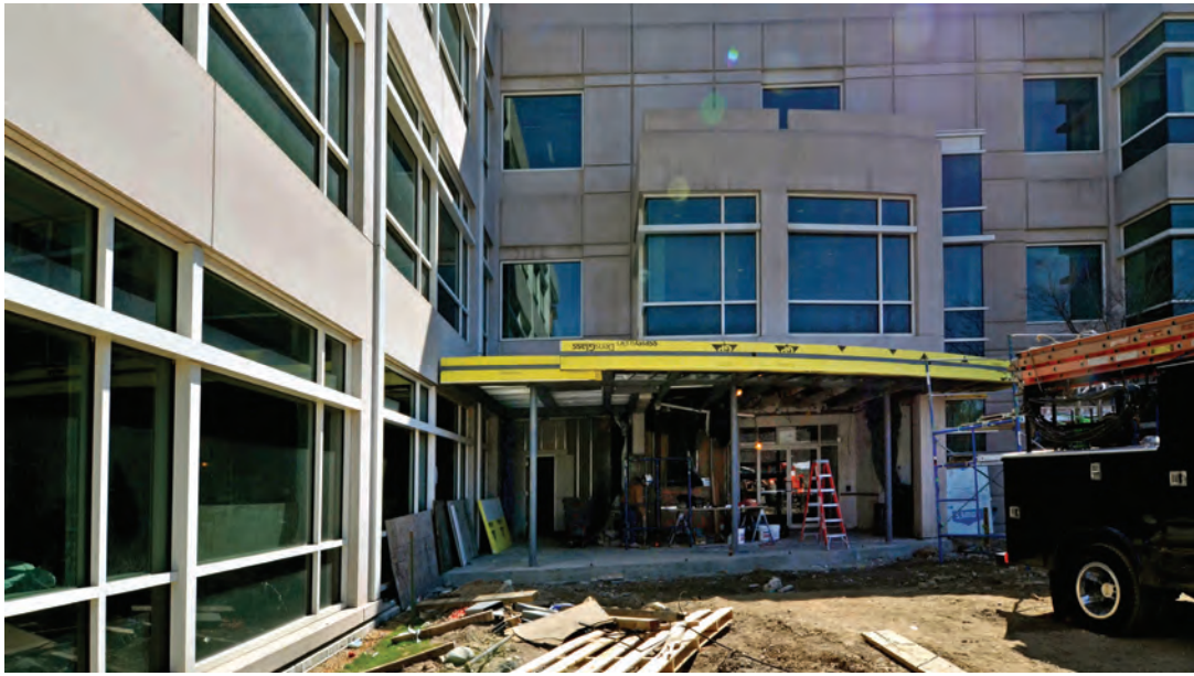
Left: Construction is underway at the new main entrance to Yale School of Nursing.
